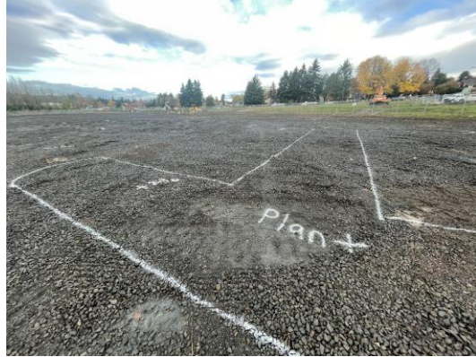
11/5/21 Parcel 2 capping demarcation.
