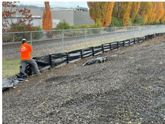
10/28/21 Silt fencing being installed on Parcel 2.
