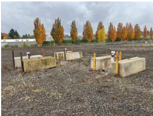
10/27/21 Parcel 2 wells protected by Ecology blocks.
