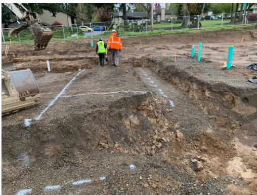
4/12/22 Building 4 footings, looking north.
