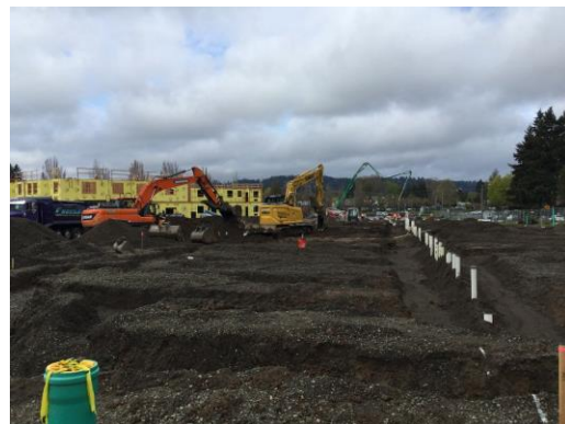
4/14/22 Building 4 footings, looking west. Building 2 slab pour in background.
