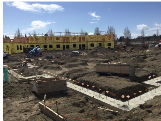
4/5/22 Building 3 footings, looking south-southwest towards Building 1.
