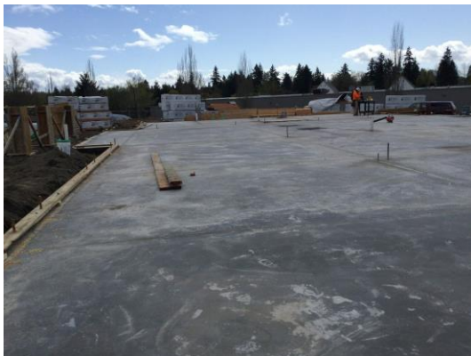
4/5/22 Clubhouse after slab pour, looking south-southwest.
