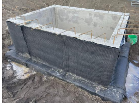
3/16/22 Stem walls after Hydroduct 220 placement, prior to backfilling.
