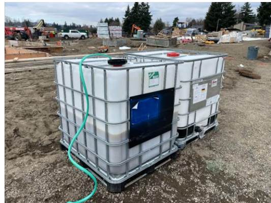
2/24/22 Stormwater pumped out from Parcel 2 Clubhouse elevator pit.
