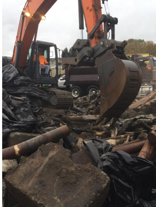
11/1/22 Parcel 2 hazardous debris haul, viewing north.
