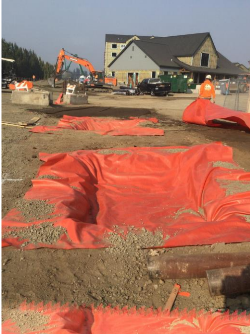
10/18/22 Parcel 2 tree well excavations with liner, viewing northwest.
