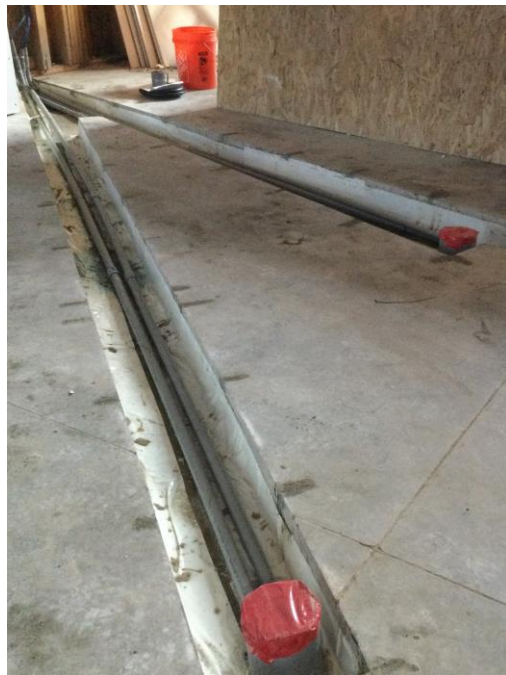
12/27/22 Parcel 2 Clubhouse completed vapor barrier repair before concrete slab pour.
