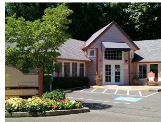
Waverley Green Apartments are installing 400 kW of solar at their complex.
