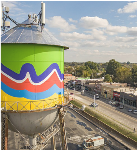
Top: Build on specific elements in the NMIA to brand the area. Bottom: Example of a branded water tower
