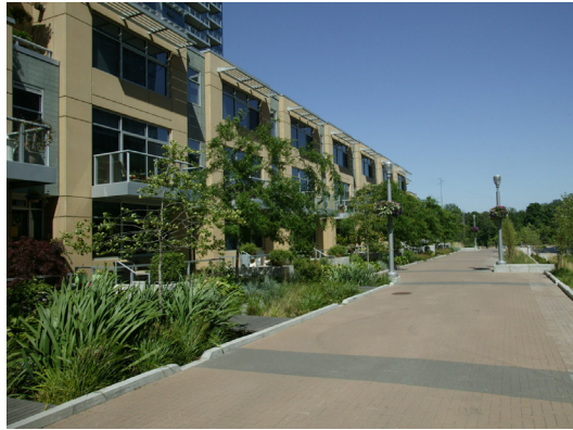
Pedestrian-oriented street with stormwater planters
