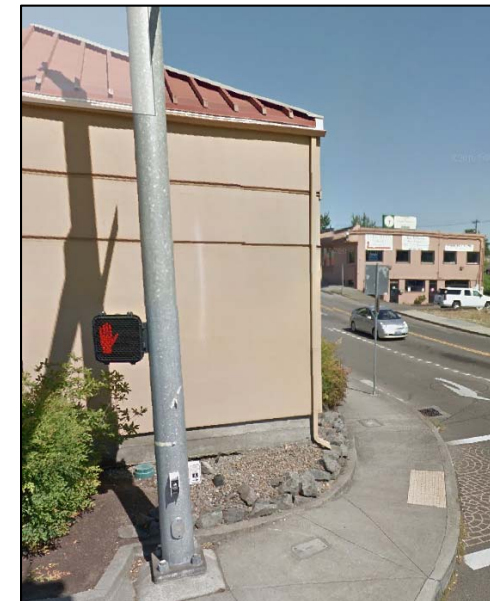
Not Recommended: Downspout drains to sidewalk (Milwaukie)
