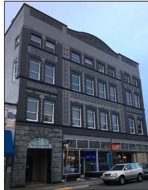
Recommended: Renovation enhances original window style and façade treatments (Masonic Lodge in Oregon City)
