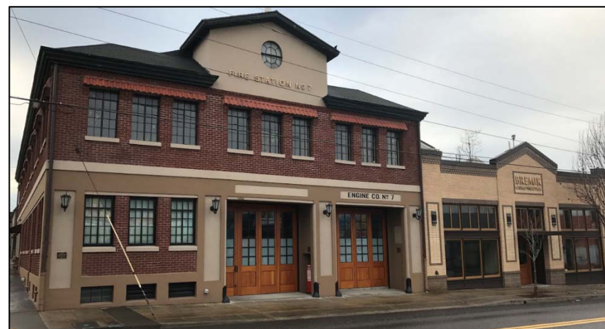
Recommended: Renovation maintains original window style and finish materials (Portland)
