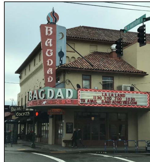
Recommended: Maintenance of original roof material, historic signage (SE Portland)
