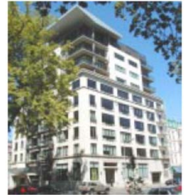
Recommended: Contemporary additions on rooftops can be compatible with the historic building if the historic facades are left intact (NW 8th and Everett, Portland)
