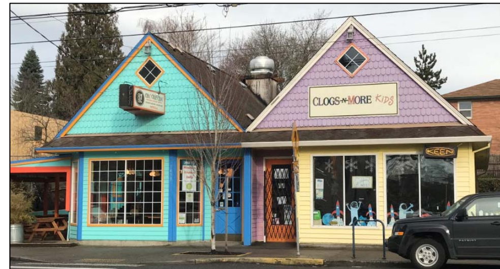
Not Recommended: Bright, varied colors and hip roof style are incongruous with surrounding buildings
