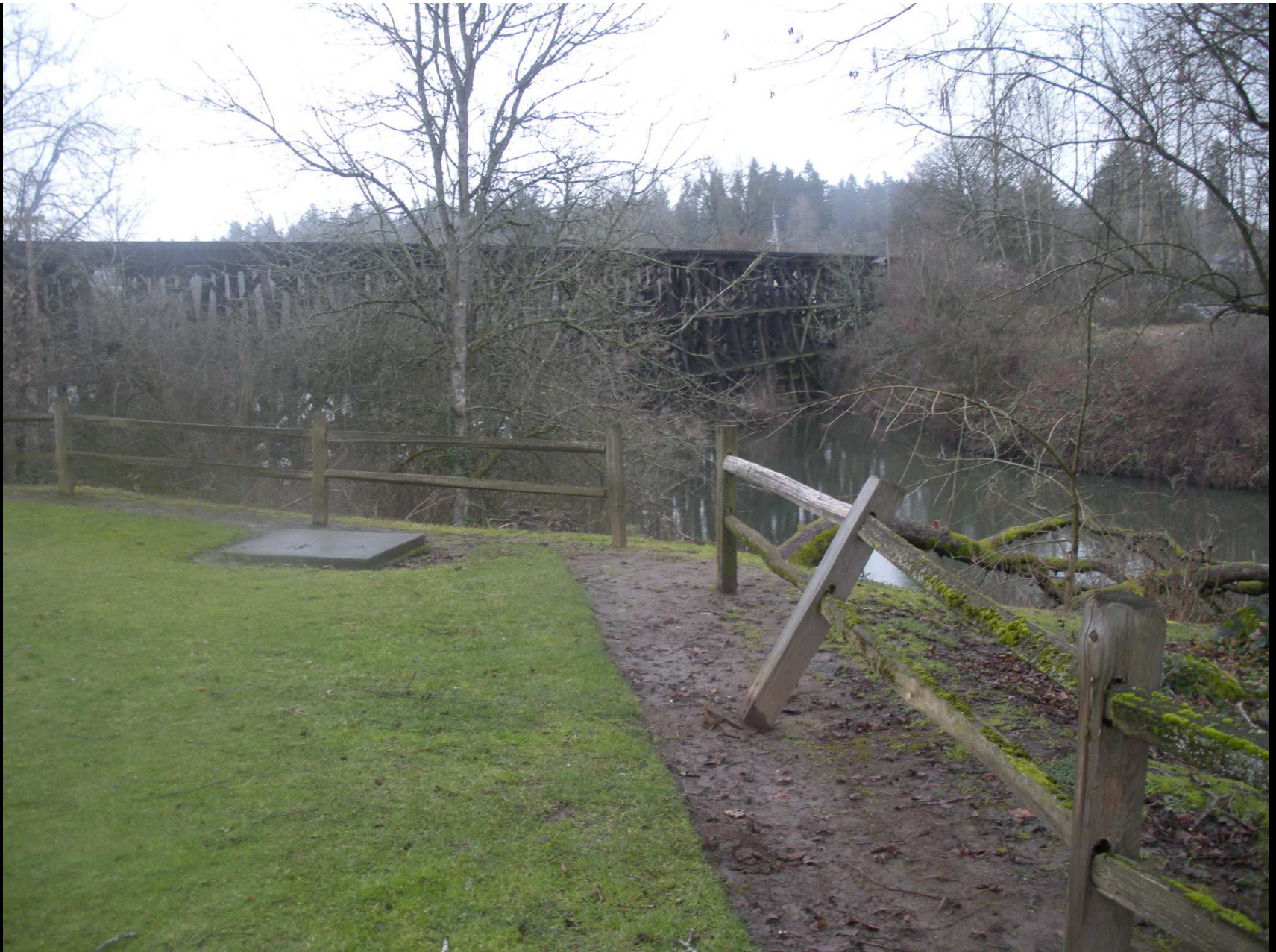
The rail trestle is a strong positive in the South Downtown
