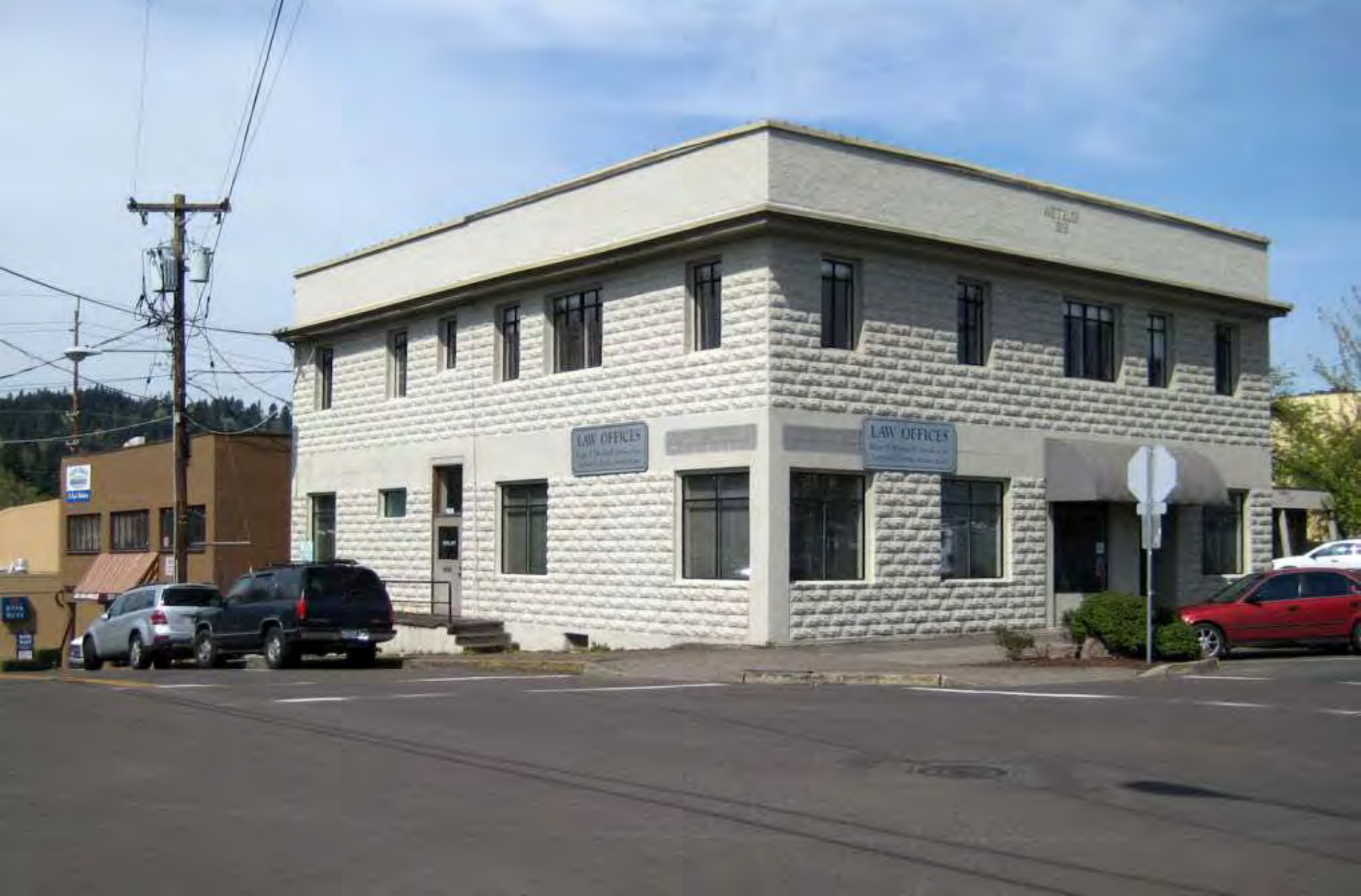
Milwaukie South Downtown: Existing Built Environment
