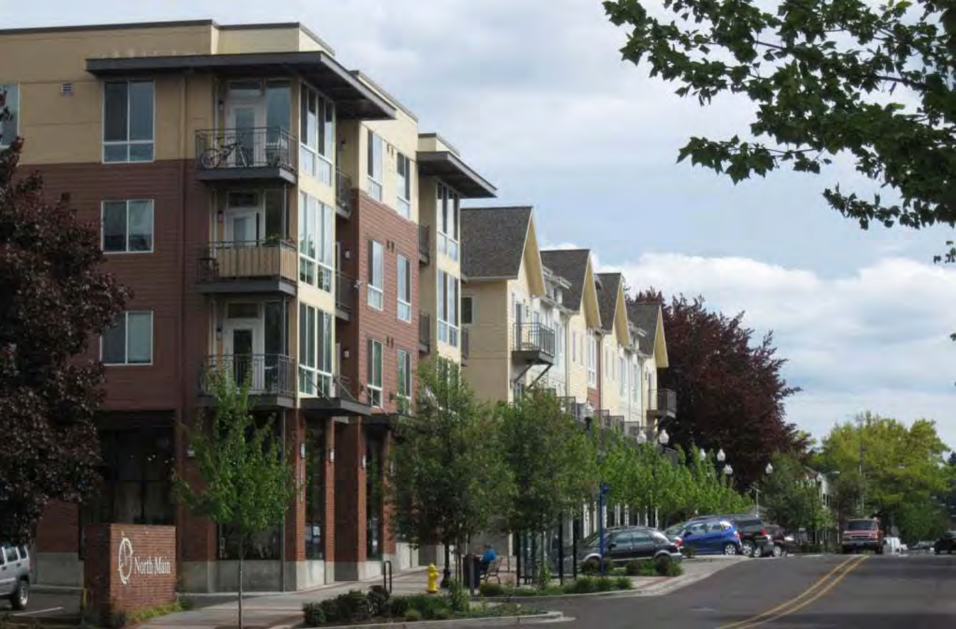
Milwaukie South Downtown: Existing Built Environment
