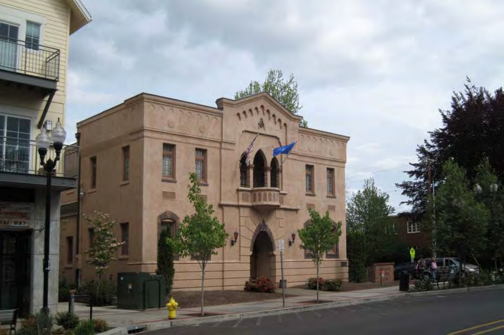
Milwaukie South Downtown: Existing Built Environment
