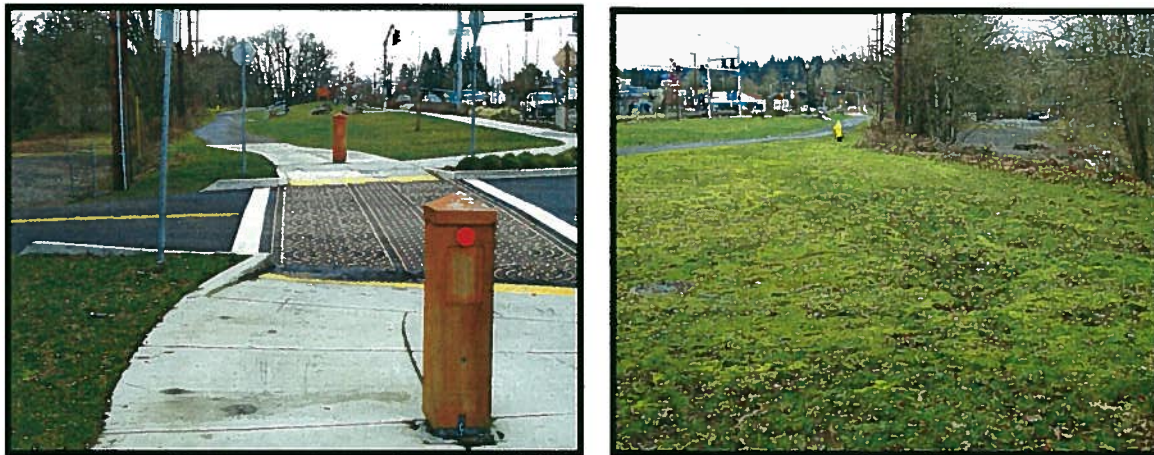
Figures 1 and 2: Area of the Portland Traction Line in Riverfront Park looking north and south, respectively.
