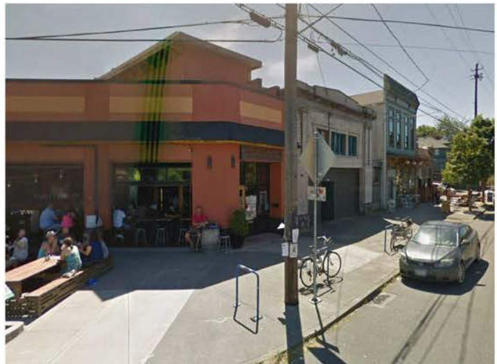
Neighborhood Hub Example: Small-scale commercial buildings clustered together surrounded by single-family homes in NE Portland.
