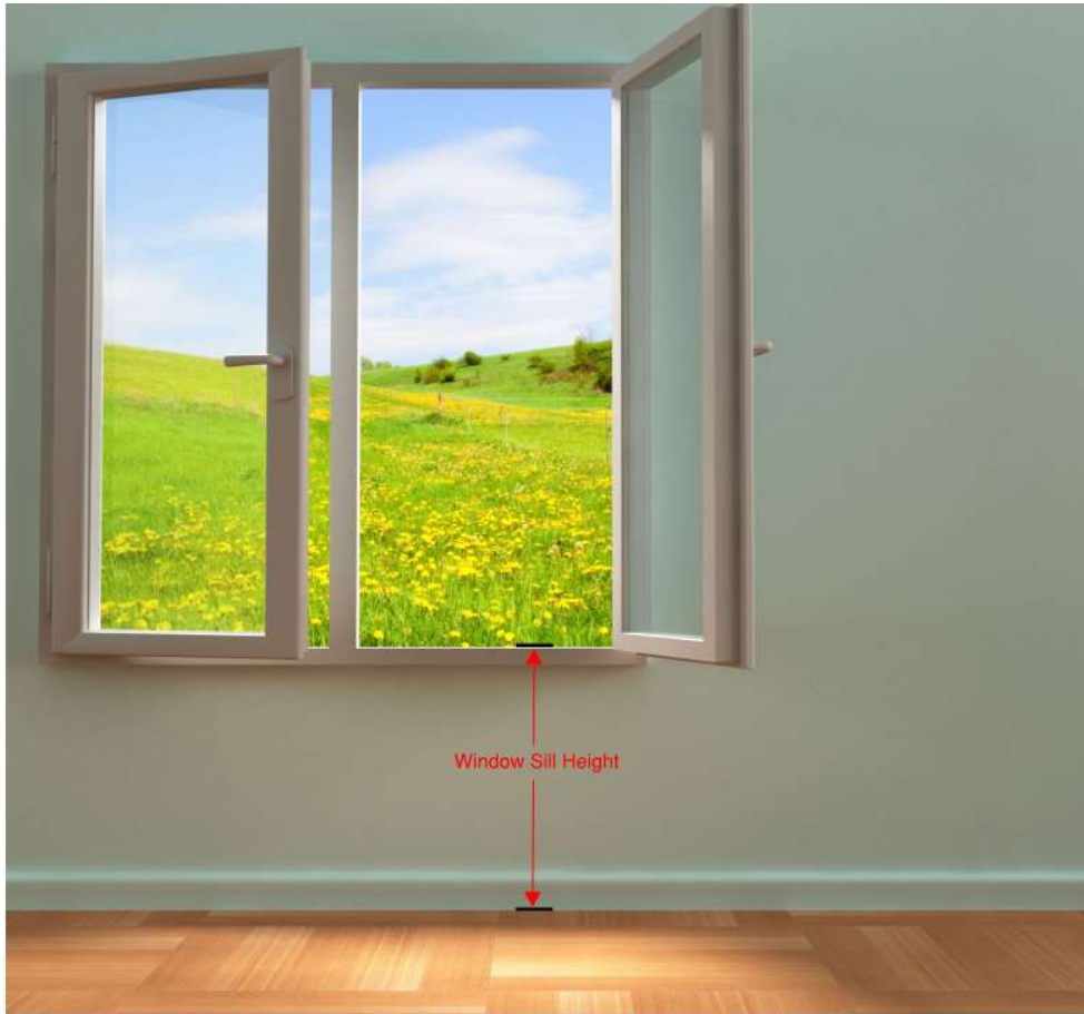
Window sill height is measured from the floor to the window opening
