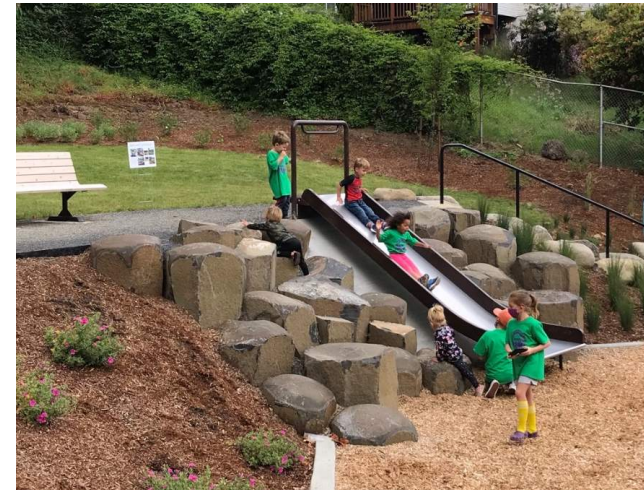
Embankment Slide: $50K Slide: $10K Boulder Scramble: $40K
