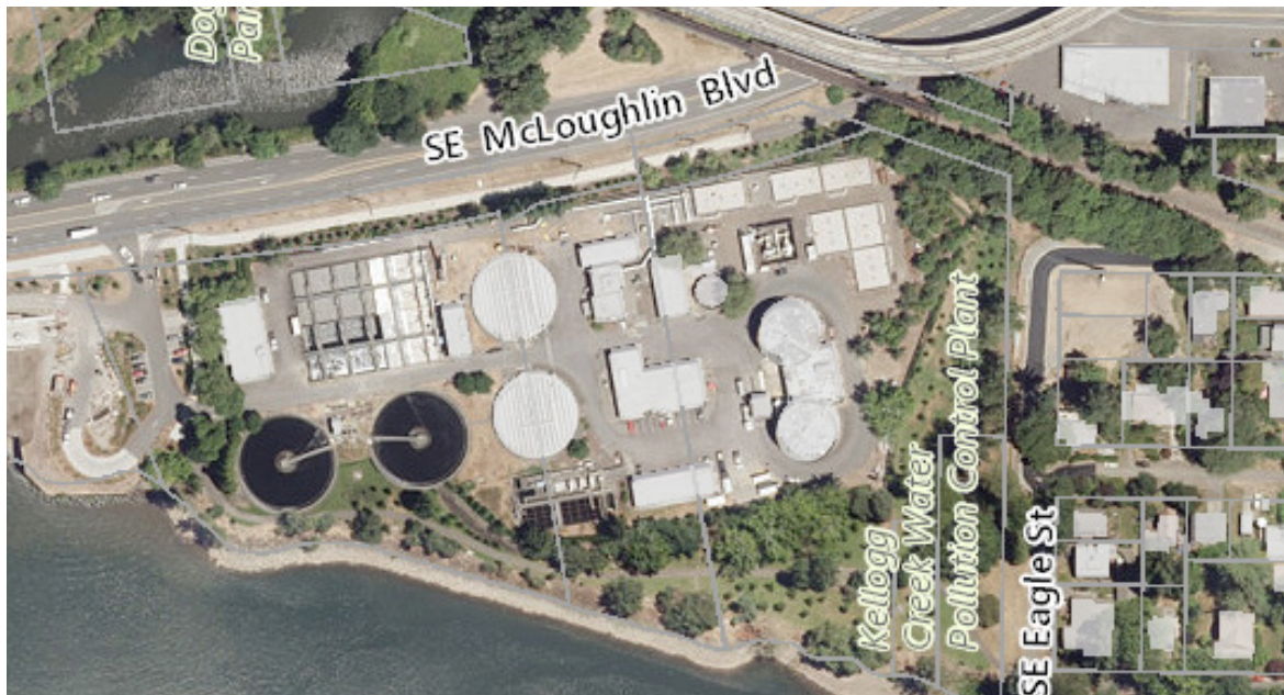
Kellogg Wastewater Treatment Plant
