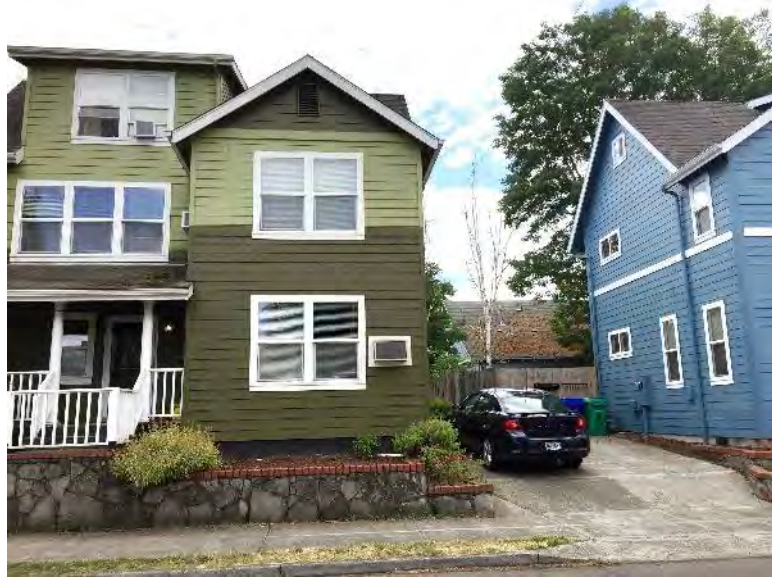
Attached housing - duplex
