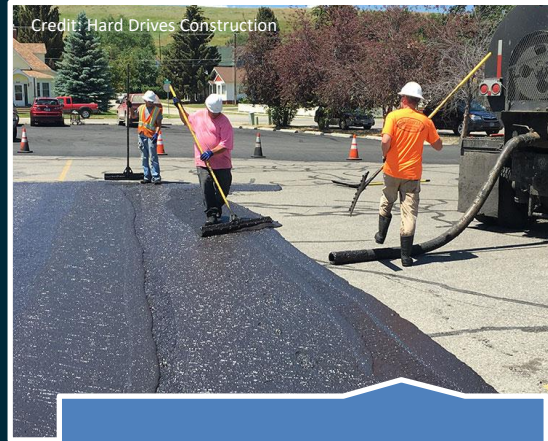
Slurry Seal
