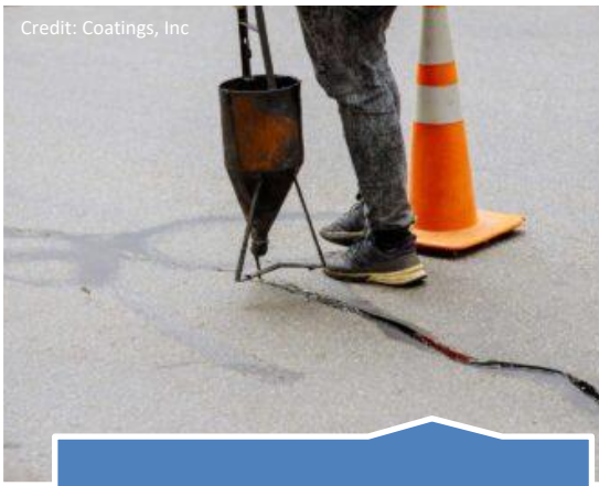
Crack Seal
