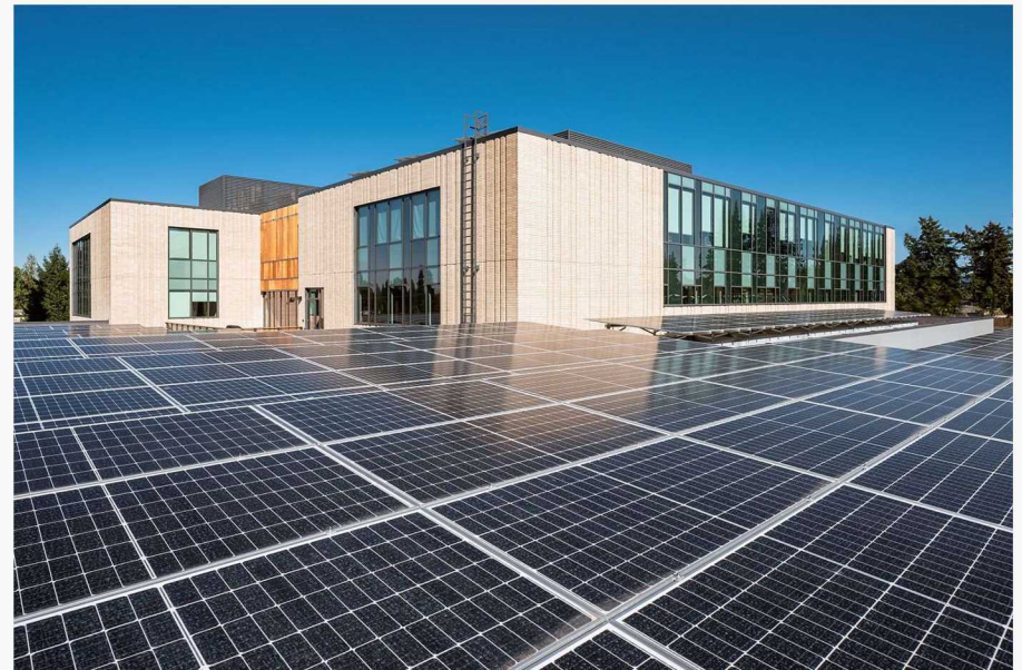
Beaverton Public Safety Center Microgrid
