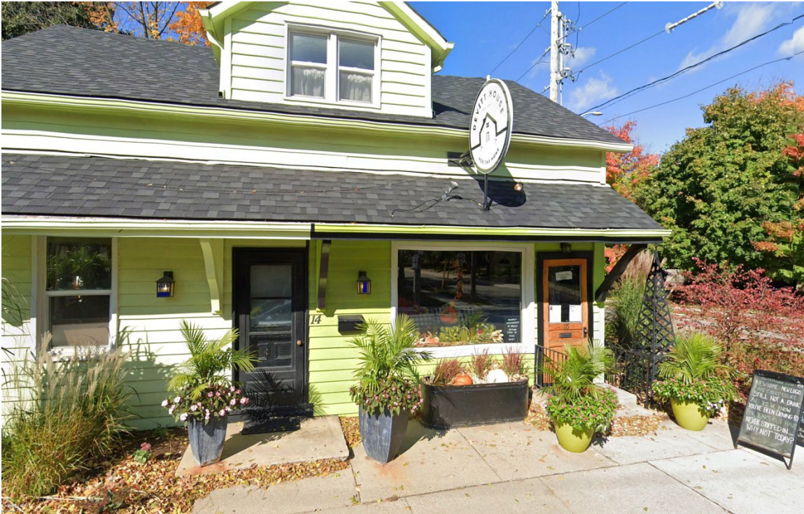
Figure 5: An ACU in Waterloo, Ontario (Photo: Strongtowns)
