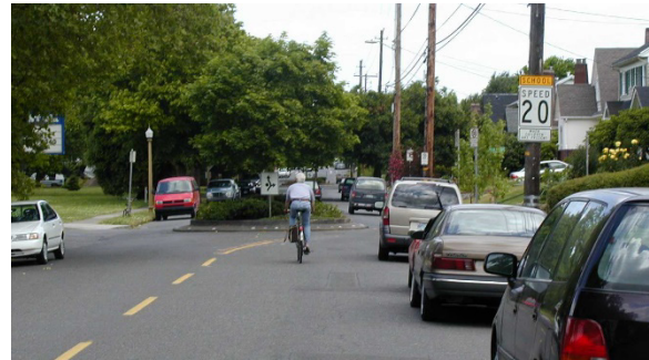
Mini circle slows traffic, creating conditions needed for shared roadway
