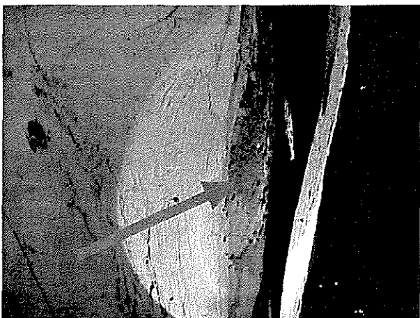
Insect damaged wood at the basement center beam support post.
