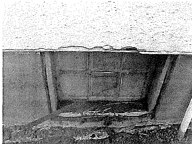
Sample of a deteriorated basement window.
