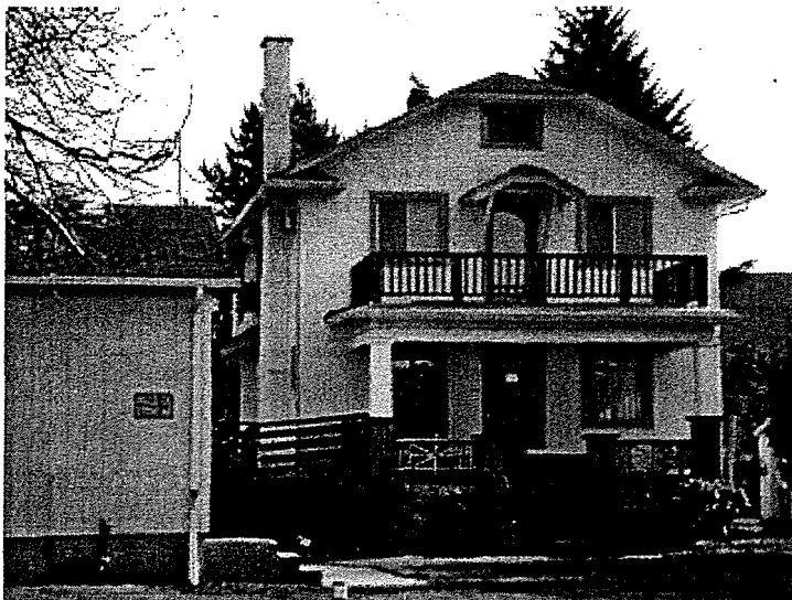
View of west facade
