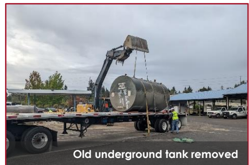
Underground fuel tank excavation at JCB
