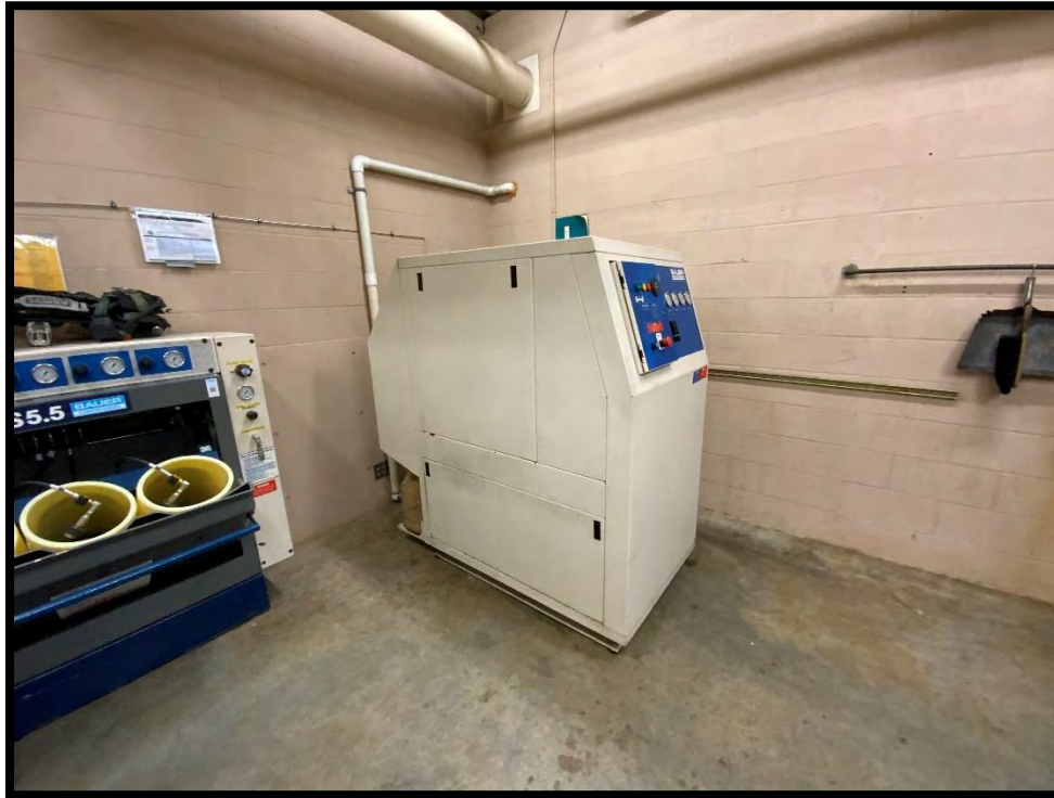
Figure 23: Example of Unraced/Unanchored Electrical Equipment
