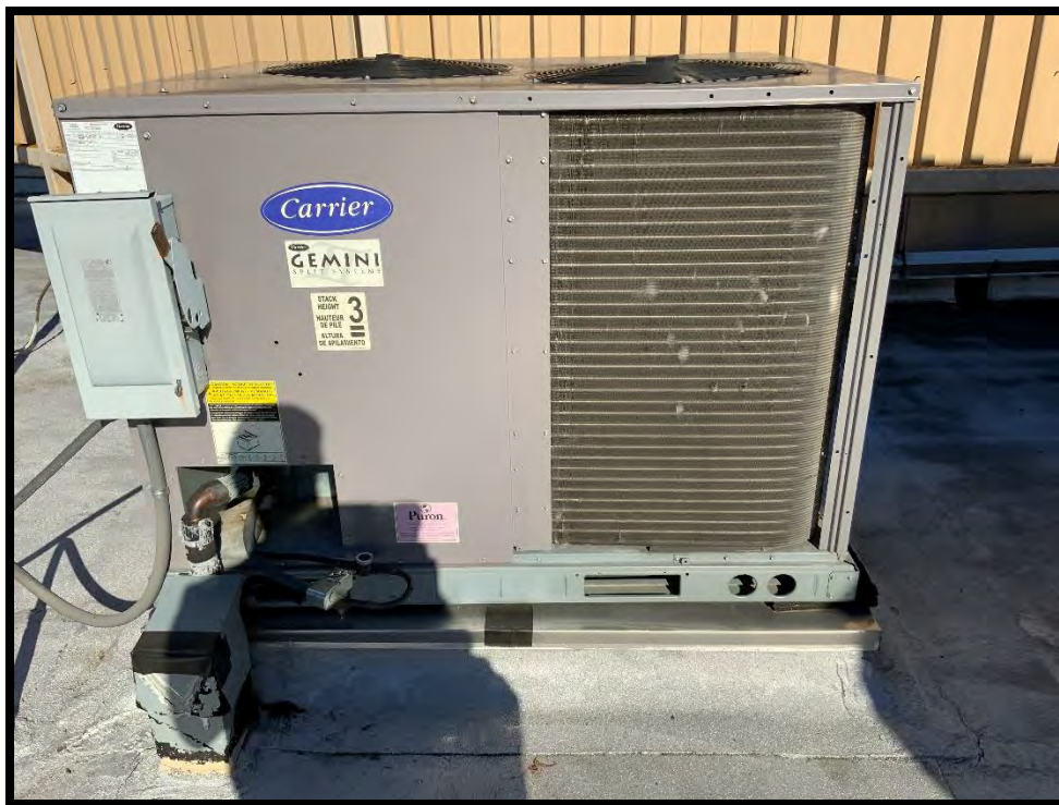
Figure 23: Example of Unraced/Unanchored Electrical Equipment
