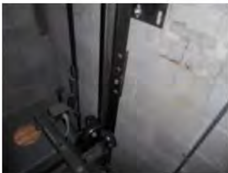
Fig. 5 – Guide rail fishplate
