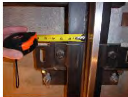
Fig. 6 – Guide rail & bracket
