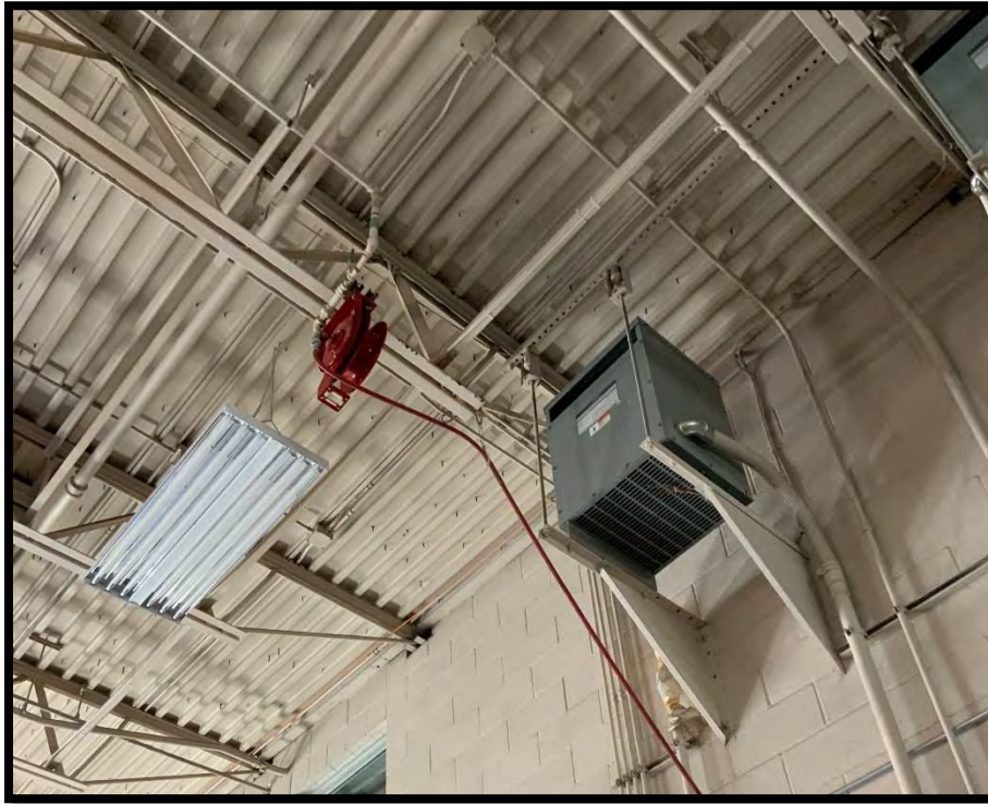
Figure 21: Example of Suspended Equipment without Sway Bracing
