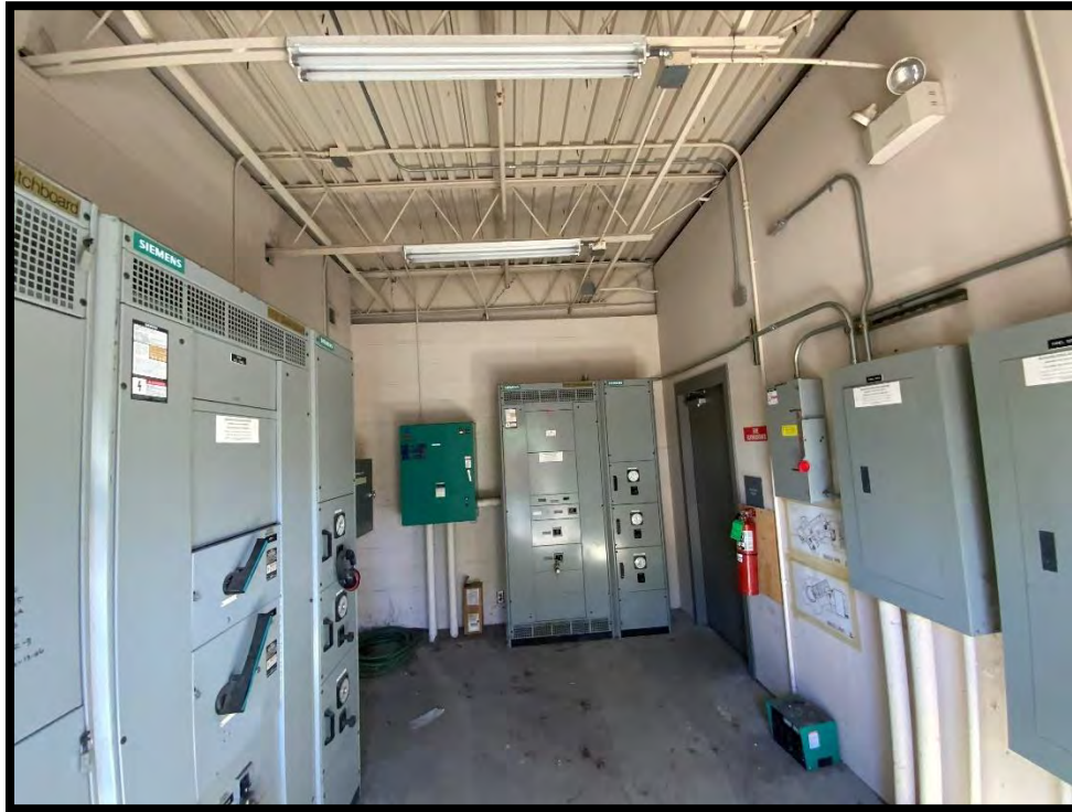
Figure 17: Example of Fall-Prone Equipment
