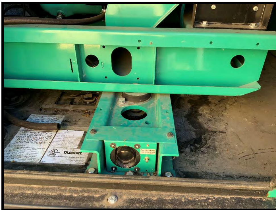
Figure 21: Example of Suspended Equipment without Sway Bracing
