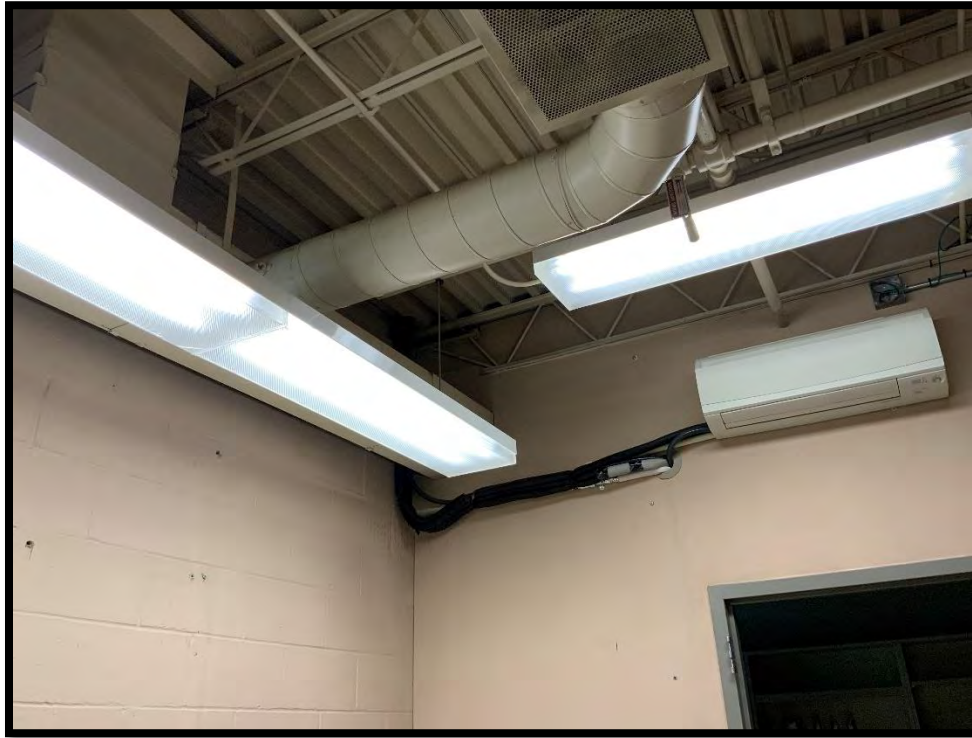
Figure 13: Example of Light Fixture Without Lens Cover Safety Devices
