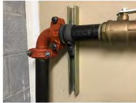
Fig. 2 – Oil line support brackets
