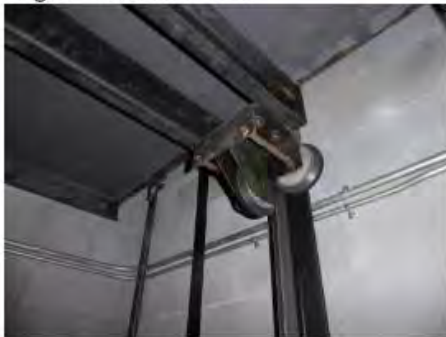
Fig. 3 – Roller guides (w/ out seismic retainer plates)
