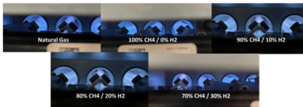
Figure 14. Visualization of condensing furnace burners at a steady state.
