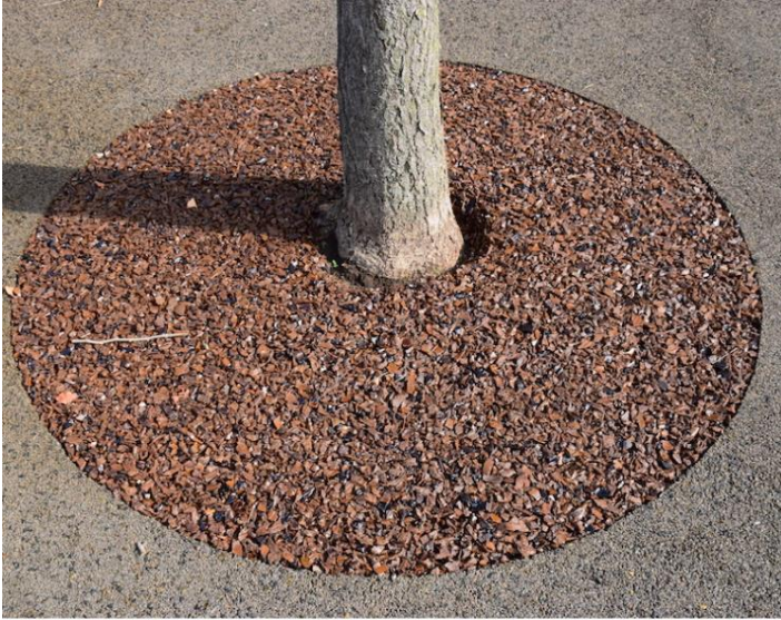
PERMEABLE TREE SURROUNDS WITH POROUS PAVE
