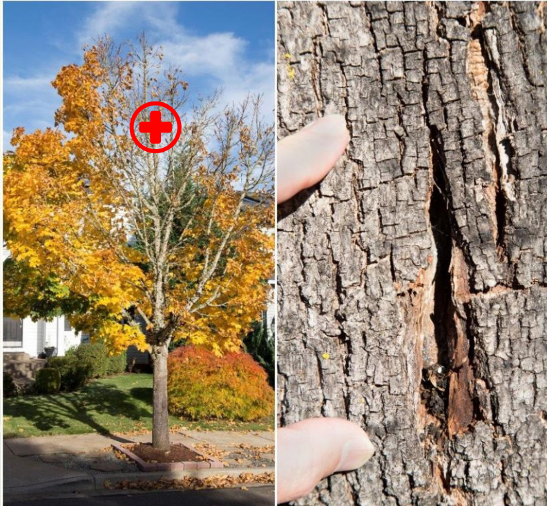
Maple tree with split from stem canker disease - unmitigable as determined by ISA arborist
