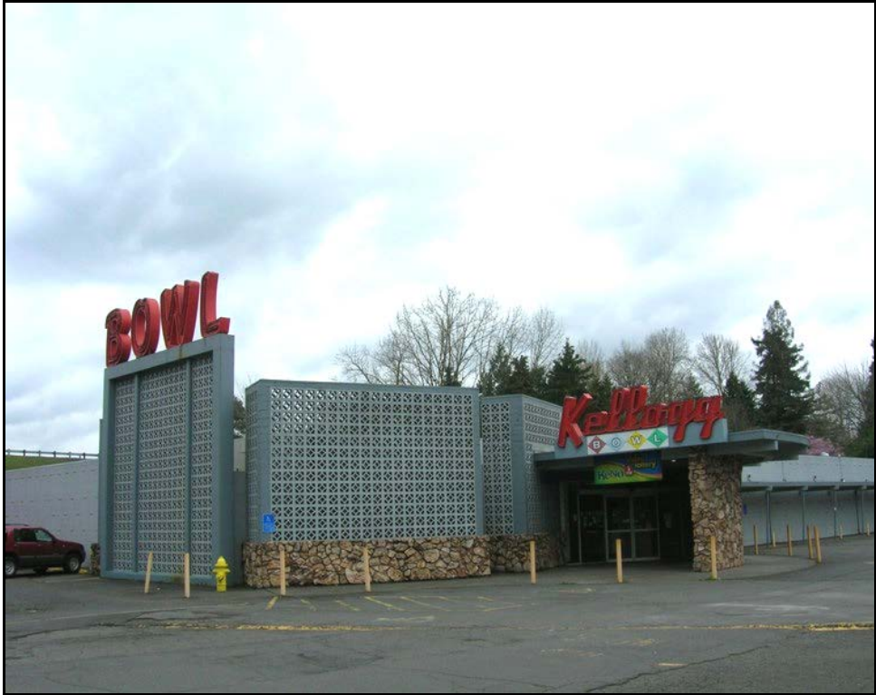
Kellogg Bowl Building (1963) at 10306 SE Main St.
