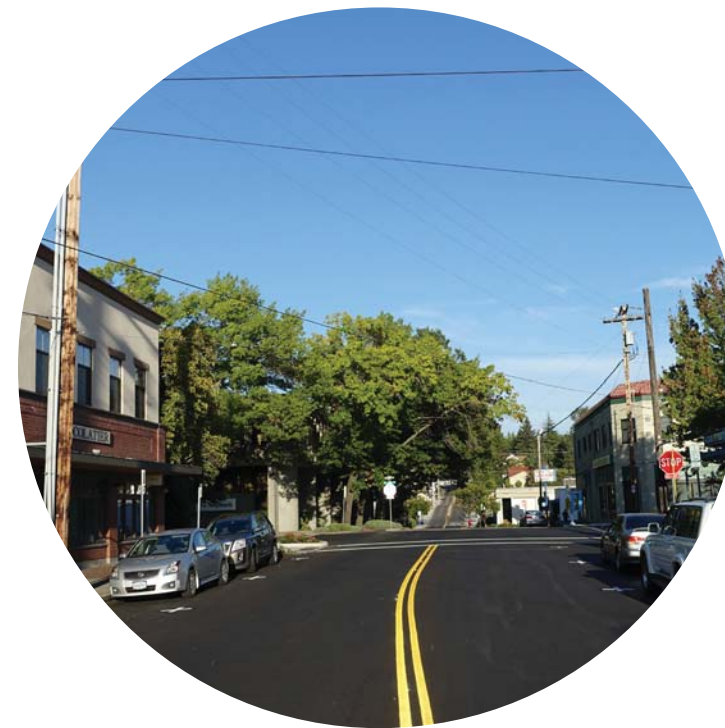
Monroe Street provides a direct link to downtown Milwaukie
