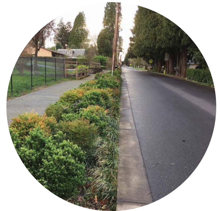
The nearby Logus Road project incorporates stormwater treatment and traffic calming features
