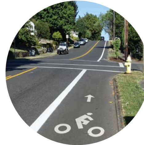
At 37th Avenue, looking east; the narrow uphill bike lane is substandard, with no downhill bicycle facility
