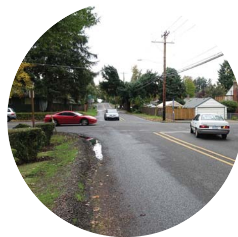
The intersection at Linwood Avenue has inadequate sidewalks, no crosswalks, and difficult sightlines
