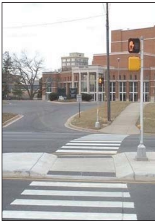
Median Refuge Island
