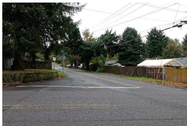
Monroe Street at Linwood Avenue (looking west) lacks sidewalks and marked crosswalks, and also features a wide curb radius
