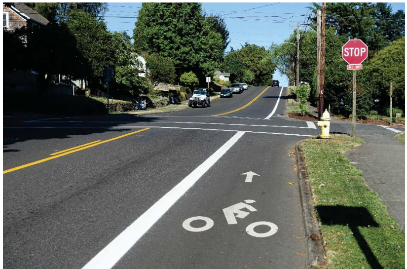
The eastbound bicycle lane narrows from 5 to 4 feet as Monroe Street climbs at 37th Avenue
