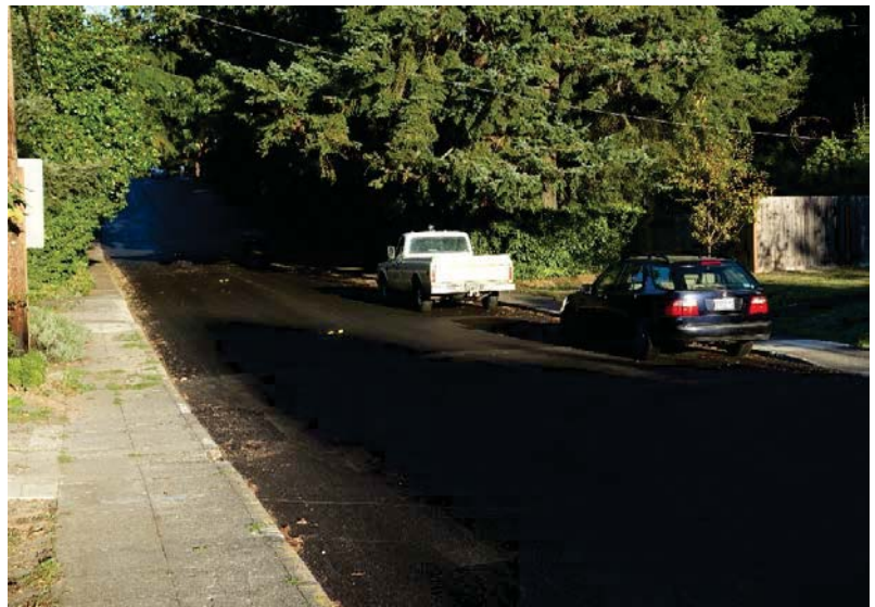
Overgrown vegetation impedes pedestrian passage on already narrow sidewalks near 28th Avenue
