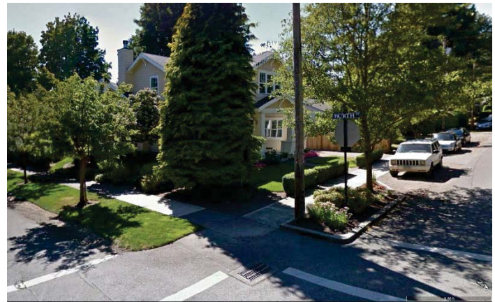
Landscaped curb extension along street without full length curb and gutter
