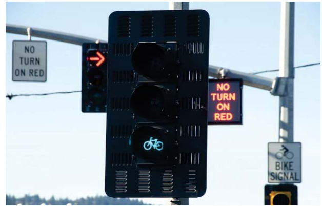
Bicycle signals help separate bicycle movements from vehicle movements at major intersections and reduce conflict (source: ODOT, 2009)
