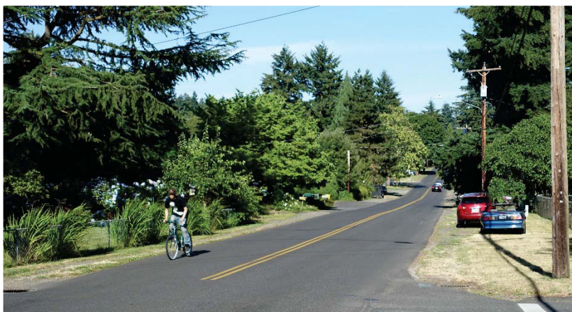
This section of Monroe Street lacks sidewalks, curbs, and gutters
