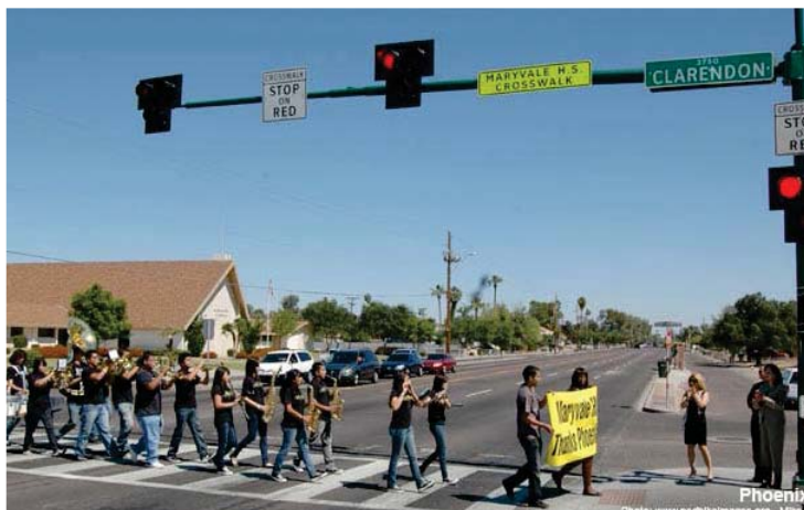
Pedestrian-activated hybrid beacons draw attention to bicyclists and pedestrians crossing the intersection
