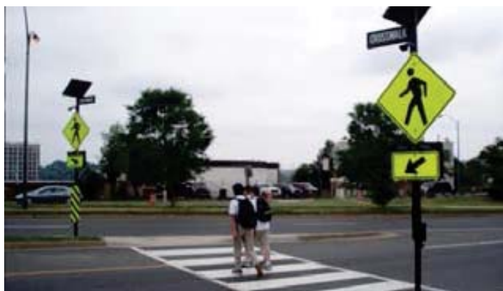
Rectangular rapid flash beacon and median island
