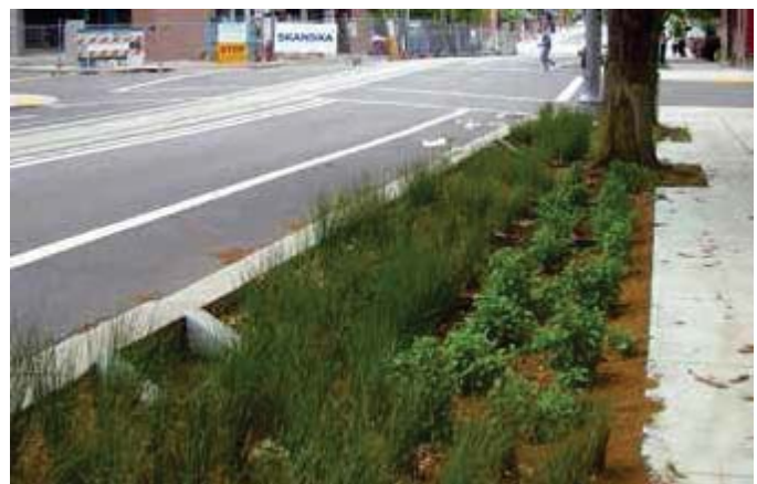
Curb extensions provide a location for landscaped swales that collect stormwater runoff
