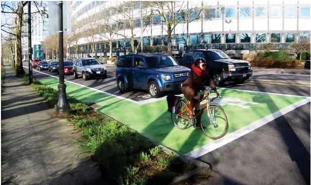
Bicycle boxes allow bicyclists to queue in front of motorists at signals to increase visibility and minimize conflicts (source: NACTO, undated)
