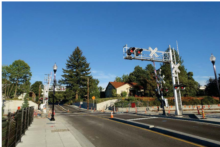
Recent sidewalk and roadway improvements around the future MAX Light Rail crossing at 23rd Avenue
