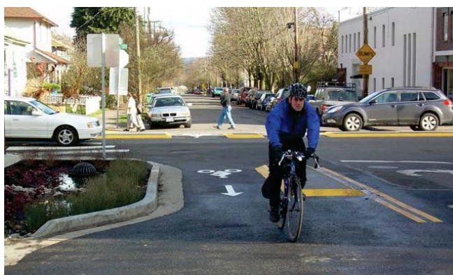
Intersection with partial diverter, curb extension, and green street features (source: NACTO, undated)
