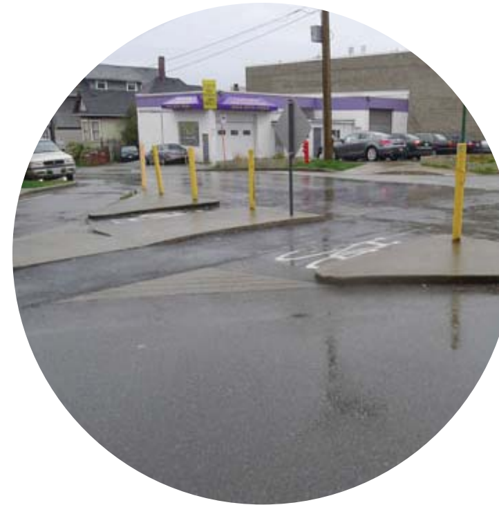
Example of a right-in/right out diverter
