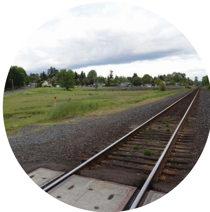
A path would run parallel to the railroad tracks through the redeveloped McFarland site
