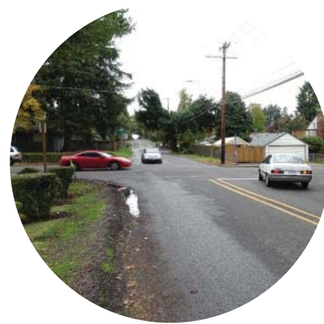
The intersection at Linwood Avenue has inadequate sidewalks, no crosswalks, and difficult sightlines
