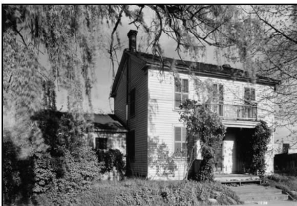
Source: History American Buildings Survey (HABS) , 1938
