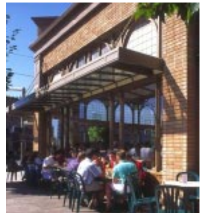
Recommended: Glass and metal canopies integrated into building facade (NE Broadway and 15th, Portland)
