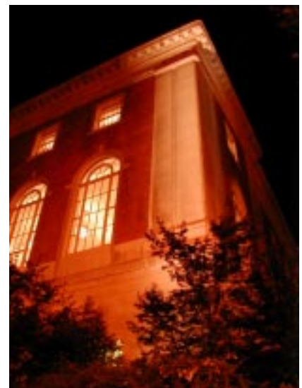
Recommended: Wall-washing light fixtures can add drama to buildings at night (SW 10th and Yamhill, Portland)
