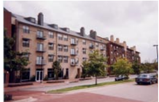
Quality affordable housing will be accessible to transit and downtown amenities.
