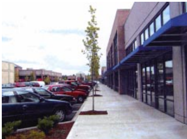
Not Recommended: Storefront windows without panels below (Teufel Village, Wilsonville)
