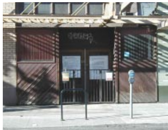
Not Recommended: Fixed security bars on windows and storefronts and security gates in front of the entrances (N Denver and Kilpatrick and NW Couch and 4th, Portland)
