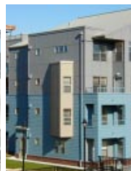
Not Recommended: Bays that are poorly detailed, clad with corrugated metal, or include projecting mechanical units (Salem Transit Center, Union Station Housing, NE Weidler and 15th, Union Station Housing)
