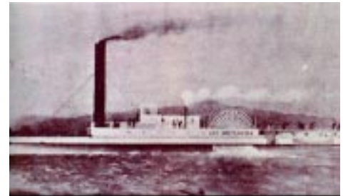
Lot Whitcomb on the Willamette River in Milwaukie, 1850.
