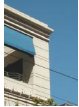
Recommended: Well articulated, deep cornices on flat-roofed buildings (SW Yamhill and 3rd, Portland)
