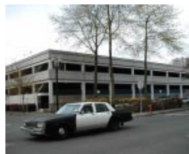
Not Recommended: Long dark horizontal openings dominate facade (NW Hoyt and 9th, Portland)
