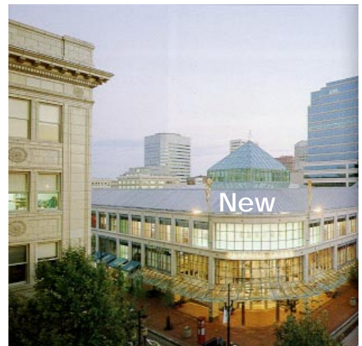
Recommended: The new building is visually linked to the adjacent historic building through the use of a similar design vocabulary ( Pioneer Place, Portland )
