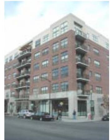
Recommended: Tripartite facade - clearly marked base, middle and top (NW 13th and Johnson, Portland)
