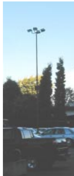
Not Recommended: Overscaled, utilitarian lights in parking lots (SW 2nd and Alder, Portland)
