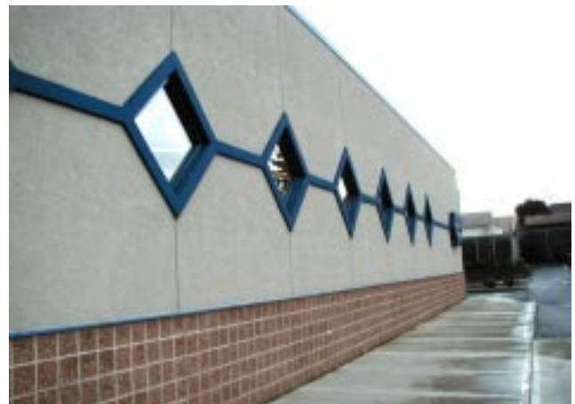
Not Recommended: Horizontal wall character exaggerated by the lack of wall definition and the oddly sized and shaped windows (N Lombard and N Denver, Portland)
