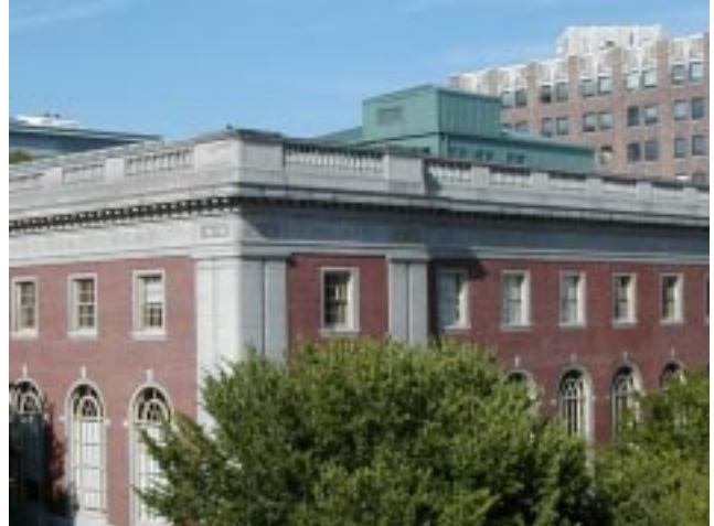
Recommended: Roof parapet that screens penthouse office beyond (SW Morrison and 10th, Portland)
