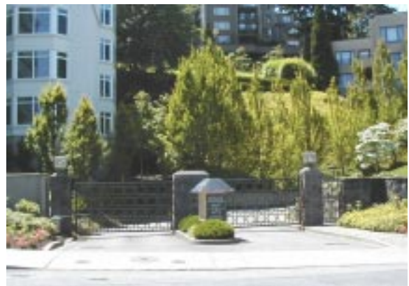
Not Recommended: Private compounds (NW Westover, Portland)
