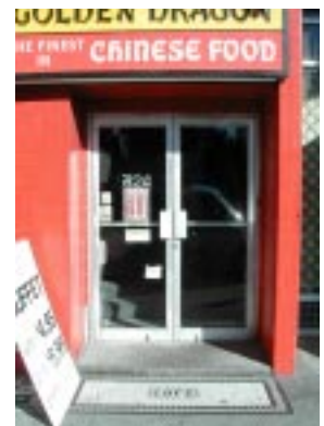
Not Recommended: Unpainted aluminum door frame (SW 3rd and Stark, Portland)
