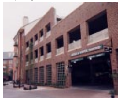
Recommended: Parking garage in scale with nearby buildings (Dallas, TX)
